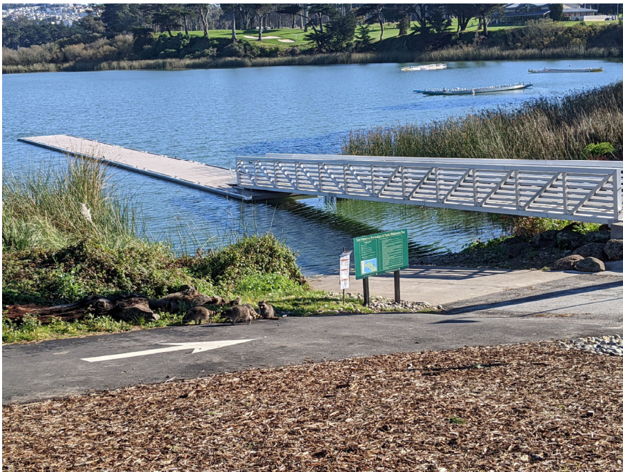
View across boat launch ramp area.
