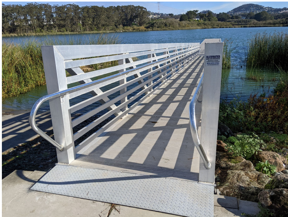
Entrance to new gangway from landside amenities leading to dock
