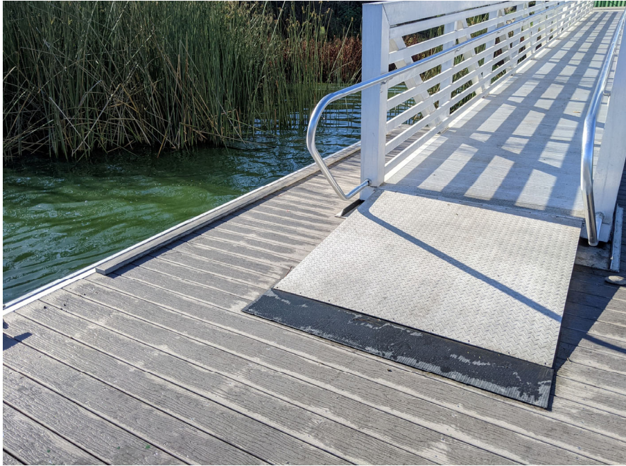
View of transition plate between gangway and ramp.
